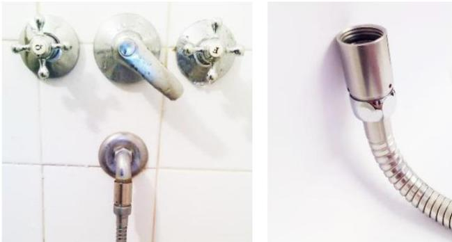
Figure 5: LowFlow® installed on the hand held shower hose (connecting it to the faucet).
